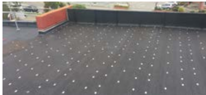
» Nuraboard mechanically fixed in place and awaiting membrane install
