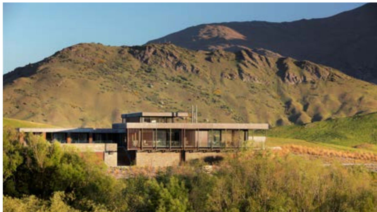
» Oliver’s Ridge by Team Green Architects
