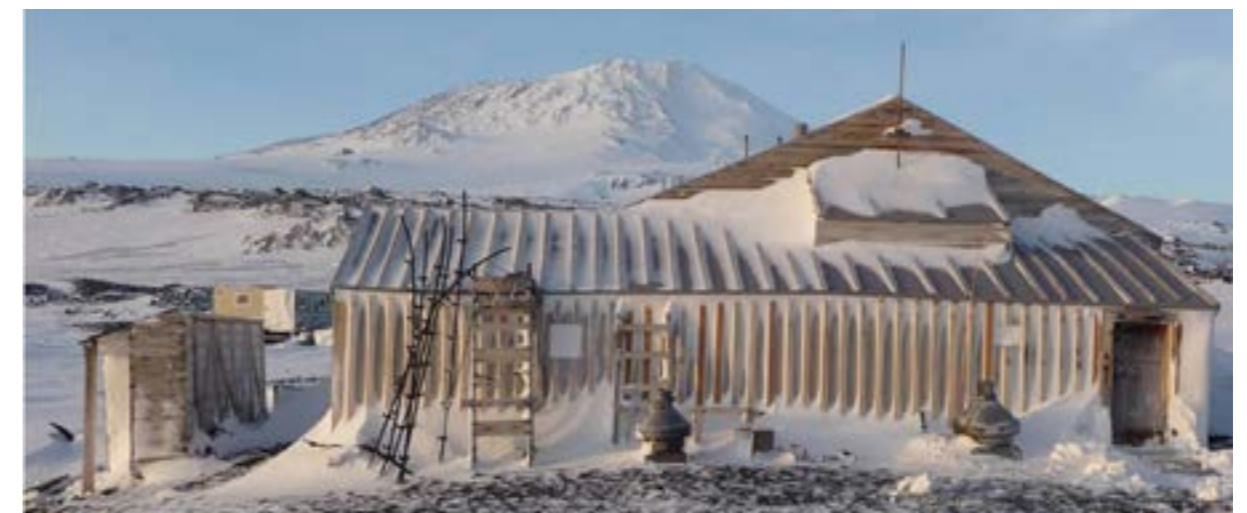
» Scott's Hut, reroofed by Cheshire Architects
