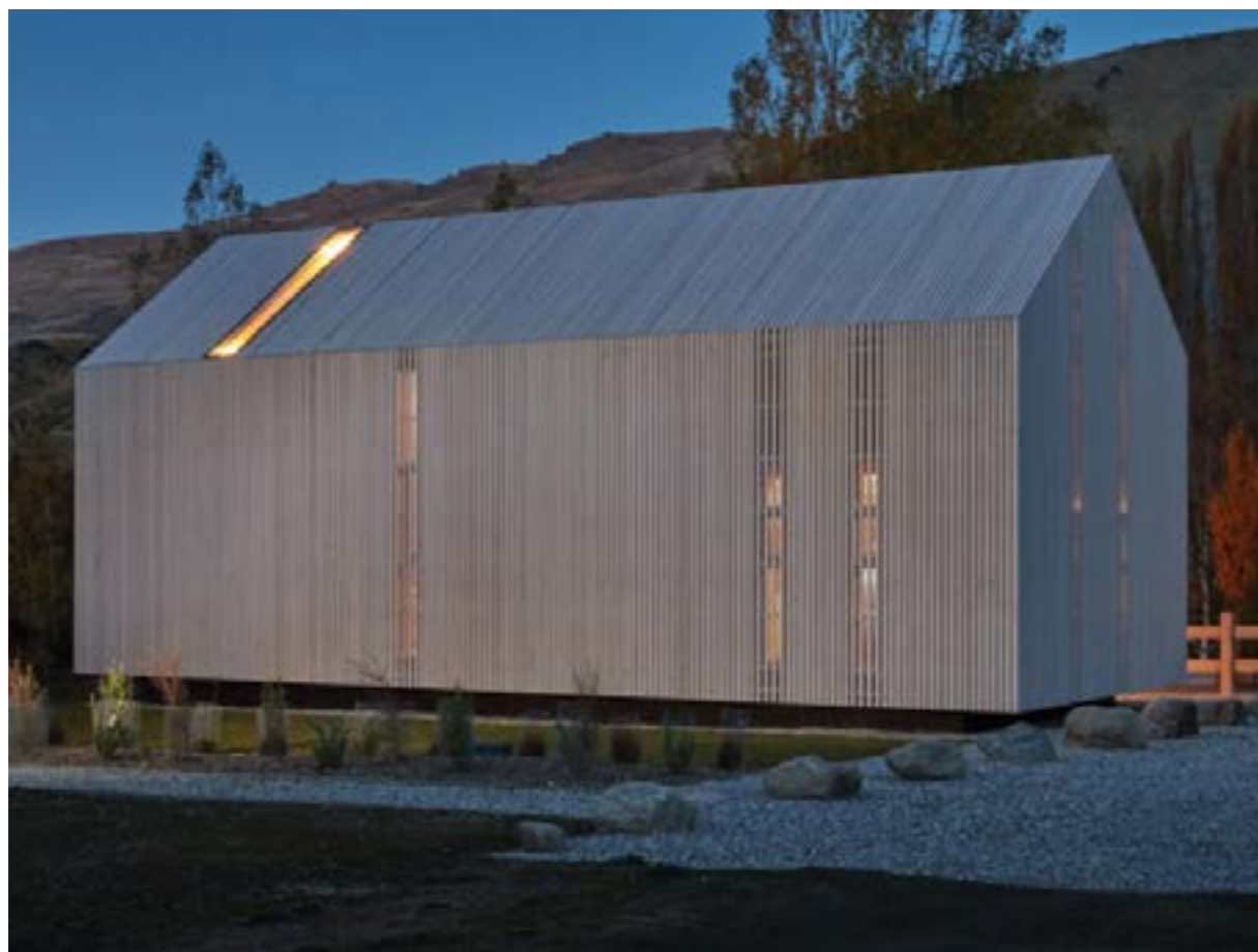
» Abodo show home By Assembly Architects. Features Nuraply membrane and Enertherm PIR insulation beneath the timber rainscreen
