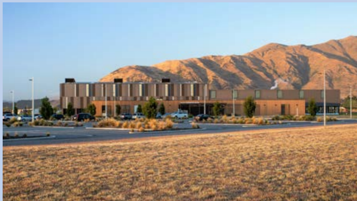
» Wanaka Sports Facility by Warren & Mahoney Architects
