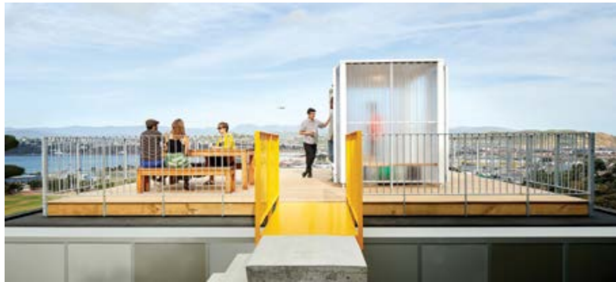
» Island floated deck by Patchwork Architects & Dorset Construction, Wellington. Nurajacks on torch-on membrane
