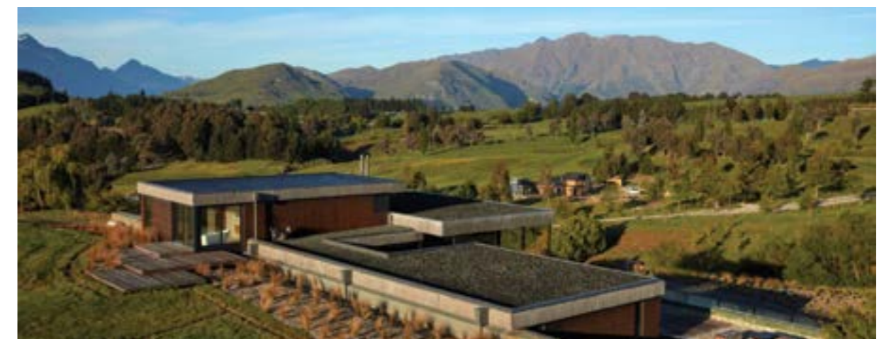
» Oliver's Ridge by Team Green Architects
