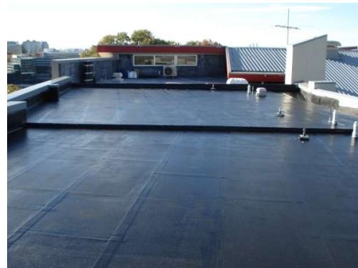
Cleaned and Primed
