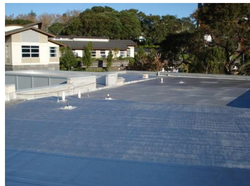
Completed overlaid roof
