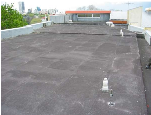
Roof in Original Condition
