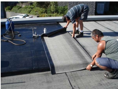
Measuring out new membrane
