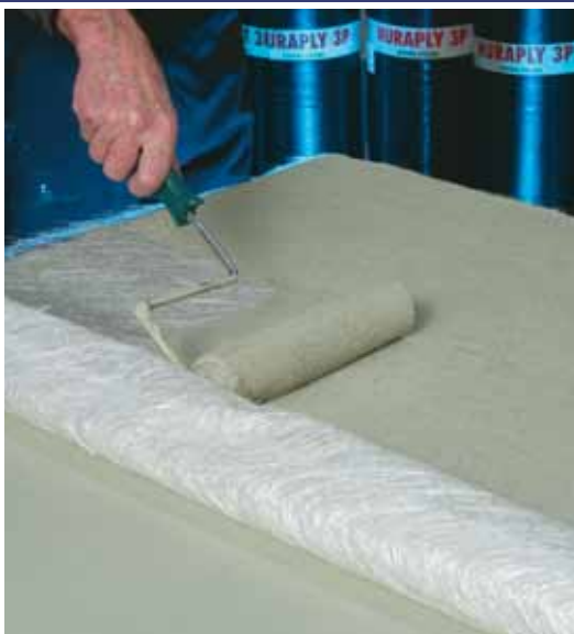
B (Nuradeck fiberglass reinforcing)
