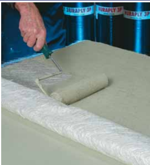
B (Nuradeck fiberglass reinforcing)
